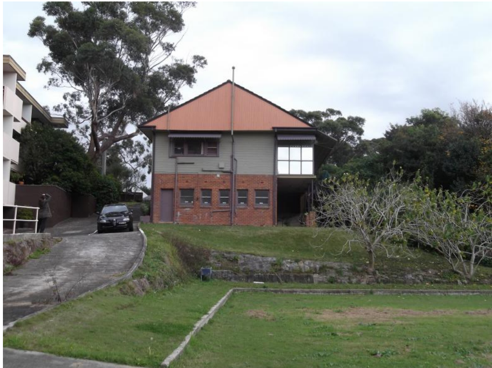
Photograph 7: Rear of existing building on site
